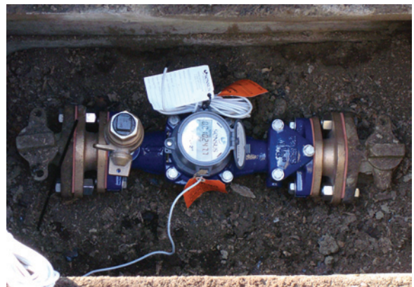
1 1/2" OMNI Meter in a 2" installation with a 2" setter showcases the ability to downsize the meter and still meet the demand requirements.
